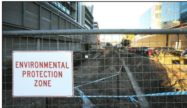
FIGURE 22: HONEYSUCKLE STATION ARCHAEOLOGY UNCOVERED IN RAIL CORRIDOR (SOURCE: NEWCASTLE HERALD, HTTP://WWW.THEHERALD.COM.AU/STORY/4037759/RAIL-RELICSCOME-TO-SURFACE-PHOTOS-POLL/ )
