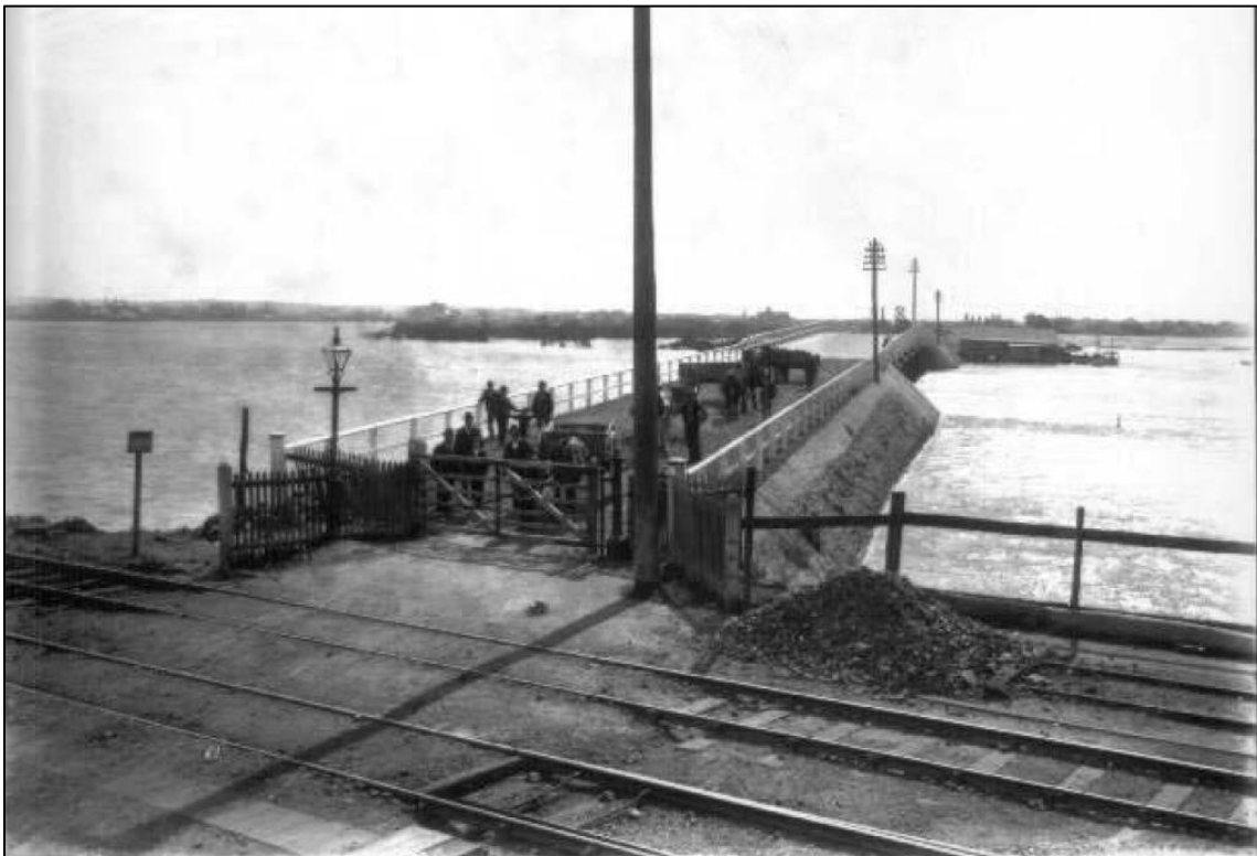
FIGURE 13: SOUTHERN CAUSEWAY OF BULLOCK BRIDGE C. 1900.
