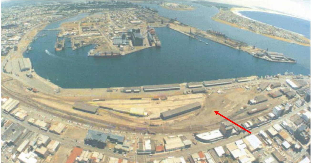
FIGURE 16: AERIAL VIEW LOOKING NORTH SHOWING THE SITE DURING PHASE 5 CLEARANCE ACTIVITY, PRIOR TO 1994 (ARROWED). SOURCE: UMWELT 2004)
